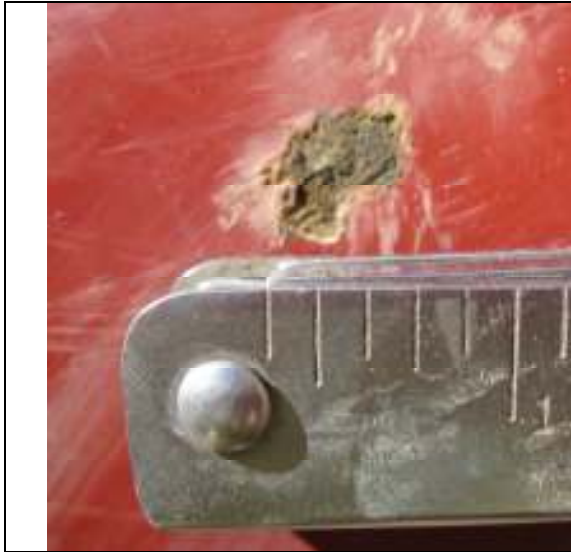
Figure 2: Small coating fault displaying evidence of burnt coating
