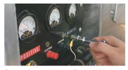
Step 10: Locate the large Red and Black wires coming from the relays in the Scout unit. To interrupt the rectifier from the negative output, remove the cable from the negative lug of the rectifier and connect the
